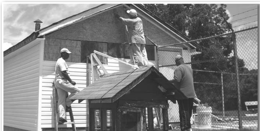
A crew puts new siding on the Helena Pool pump house. This completed the third project at the city pool —a new pool house, the conversion of the old pool house into a pavilion, and the pump house.
